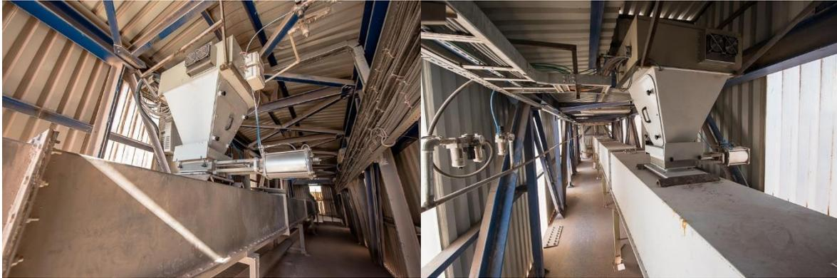
*Fig 2: The SpectraFlow Analyzer after the Raw Mill at Kiln Line 1*
